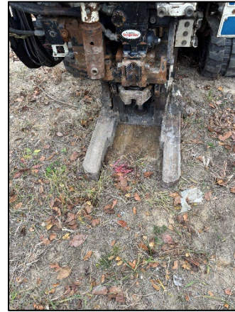
Photo 2: Viewing 8225 SB01 Drilling, Facing North.
