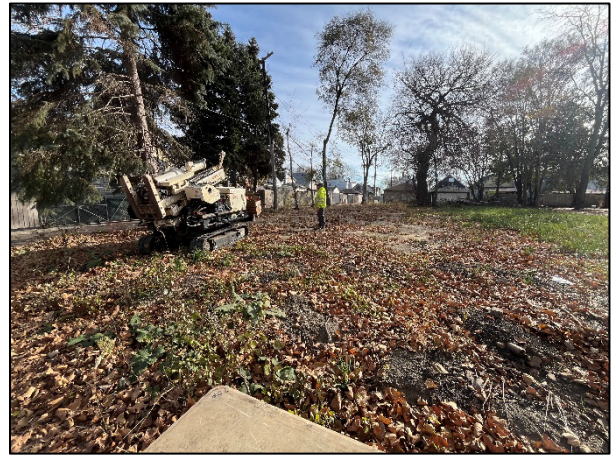
Photo 2: View of drilling activities
