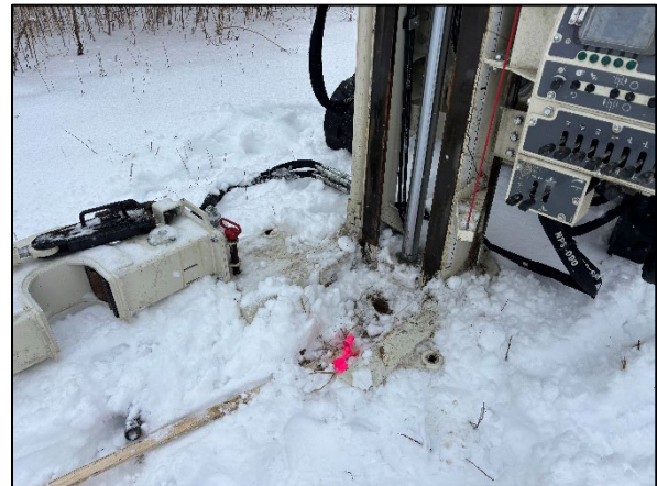
Photo 4: View of 4821 SB02, facing southwest.
