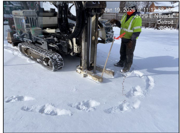
Photo 2: View of drilling at 3729 SB01, facing northwest.
