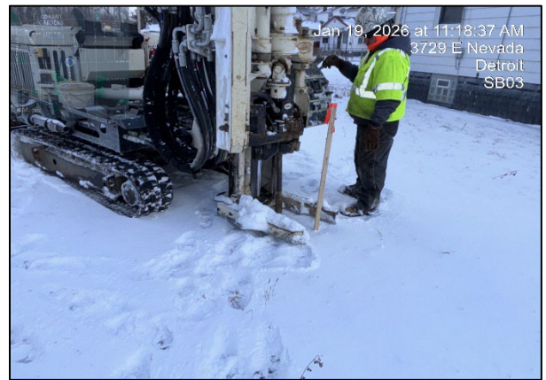
Photo 4: View of drilling at 3729 SB03, facing northwest.
