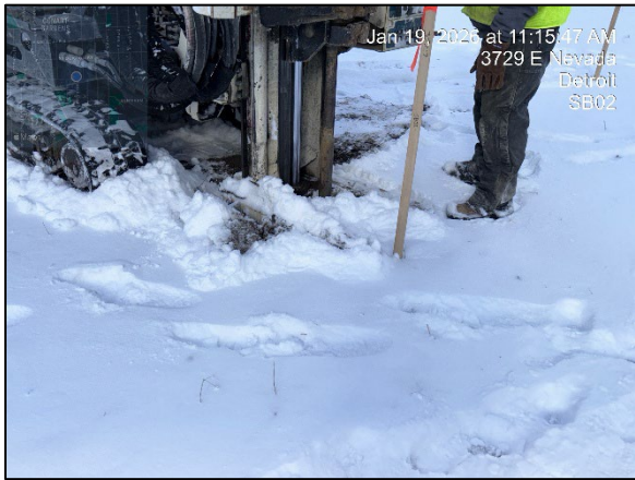
Photo 3: View of drilling at 3729 SB02, facing northwest.
