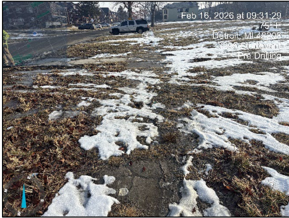
Photo 1: View of the Site pre-drilling, facing east.
