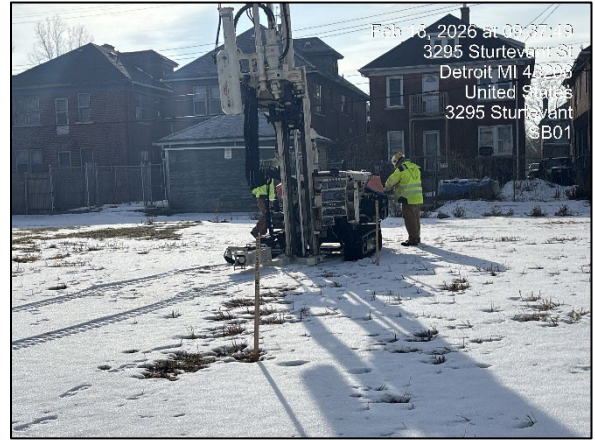
Photo 2: View of drilling at 3295 SB01, facing south.
