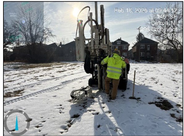
Photo 4: View of drilling at 3295 SB03, facing southeast.
