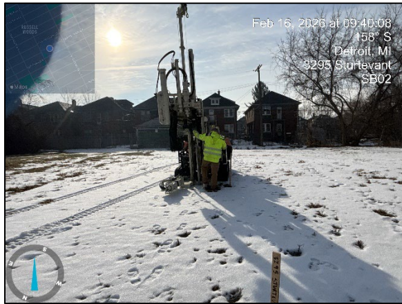
Photo 3: View of drilling at 3295 SB02, facing south.
