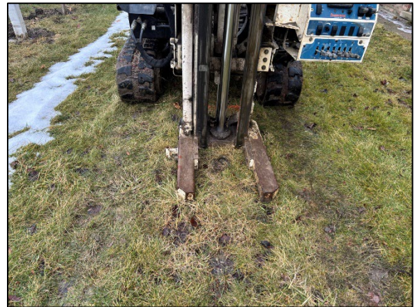
Photo 4: View of drilling at 1888 SB02, facing southeast.
