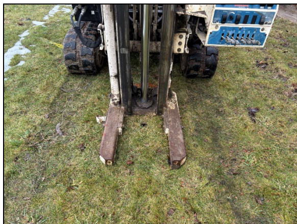
Photo 5: View of drilling at 1888 SB03, facing northwest.
