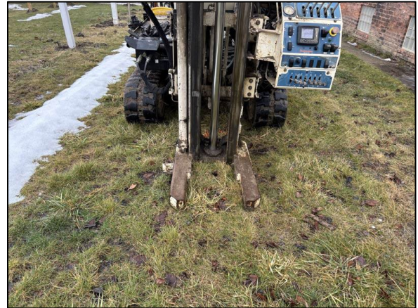
Photo 2: View of drilling at 1888 SB01, facing southeast.
