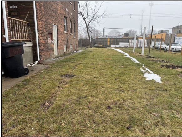
Photo 1: View of the Site pre-drilling, facing northwest.
