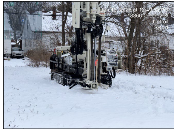
Photo 2: View of drilling at 18866 SB01, facing east.
