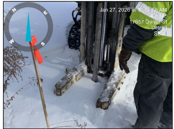
Photo 2: View of drilling at 17657 SB01, facing northwest.
