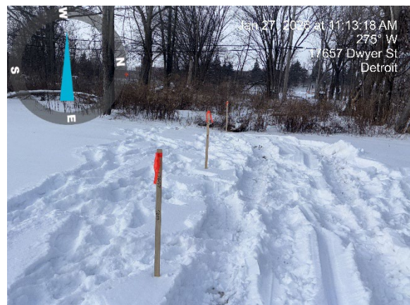
Photo 6: View of the site post-drilling, facing west
