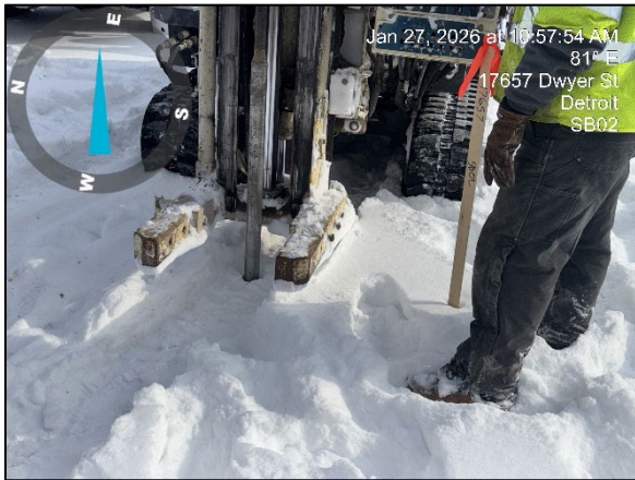
Photo 3: View of drilling at 17657 SB02, facing east.
