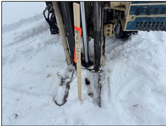
Photo 3: View of drilling 12722 SB02, facing south.
