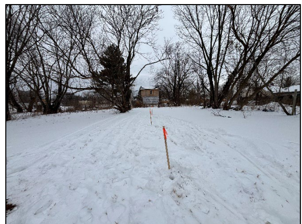
Photo 6: View of the Site post-drilling, facing northeast.
