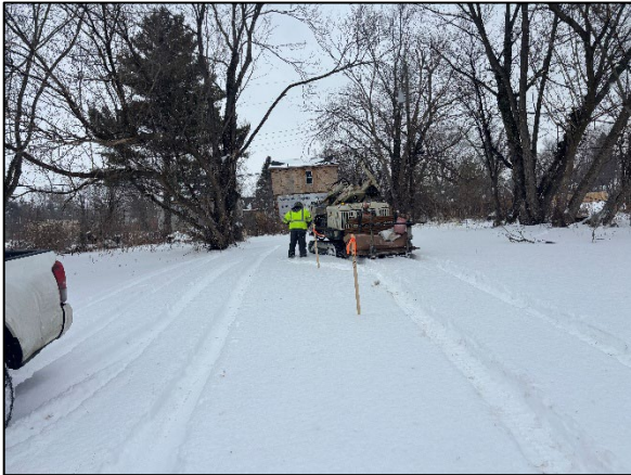
Photo 1: View of the Site pre-drilling, facing northeast.
