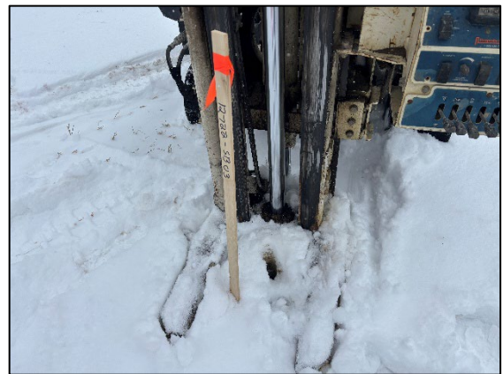
Photo 4: View of drilling at 12722 SB03, facing south.
