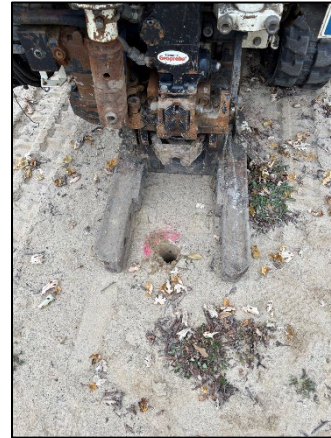
Photo 2: Viewing 12277 SB01 Drilling, Facing Northwest.
