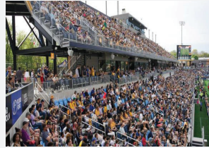
Centreville Bank Stadium, Rhode Island FC
