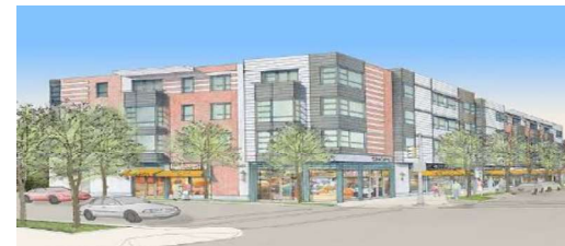
New Pennley Place: 2010- 2011 The Community Builders & PHA LIHTC 11,000 SF Retail 54 mixed-income units
