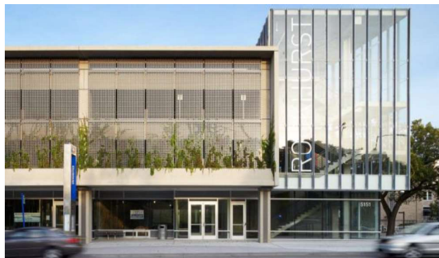
Rockhurst Retail: 2012 $9M 10K SF retail, 423 space parking garage, public plaza
